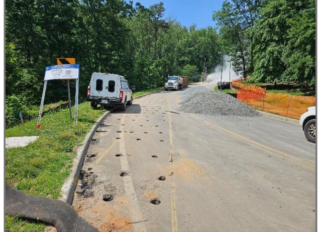
Construction on Hereford Drive – “honeycombing” process for rock removal.
