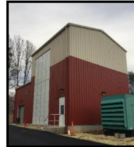
North Rivanna WTP
