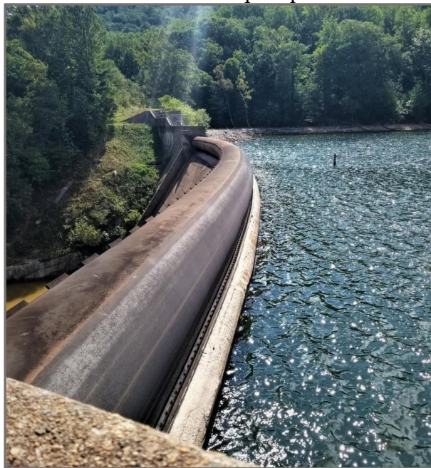
Sugar Hollow Dam Rubber Crest Gate
