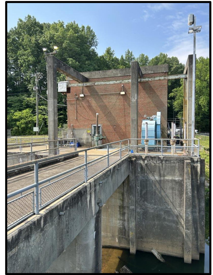
South Rivanna Raw Water Pump Station
