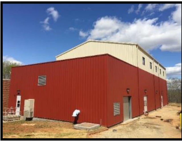
South Rivanna WTP
