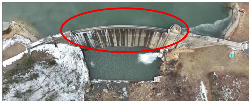
Sugar Hollow Dam Rubber Crest Gate
