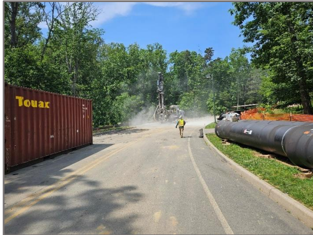
Construction on Hereford Drive – “honeycombing” process for rock removal.
